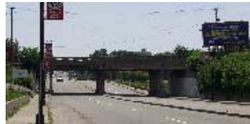
The Central Avenue Railroad Underpass
